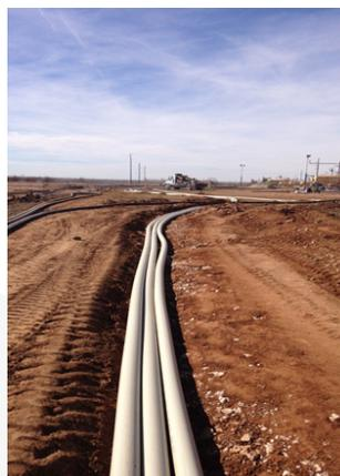
The poly pipe couldn't handle the higher pressures the wells were coming in with, and they wanted the corrosion resistance that steel couldn't provide. They installed trenched 4" FP301 HT for oil/gas/water flow lines from 6 new wells to a central header for gathering.
