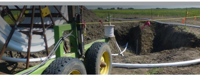
trench construction is not feasible or will cause adverse disturbances to environmental features, land use or physical obstacles. HDD installations involve drilling a pilot hole, expanding the pilot hole by reaming, and pulling back Flexpipe. Up to 2,000 meters (6,500 feet) can be pulled continuously at a time. These advantages helped the customer lower installation costs and reduce environmental impact when compared to steel.
