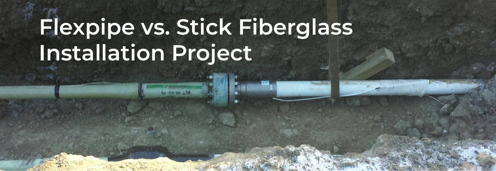
**In a side-by-side comparison, Flexpipe Linepipe provided a 20% savings in total installed cost over stick fiberglass.**
