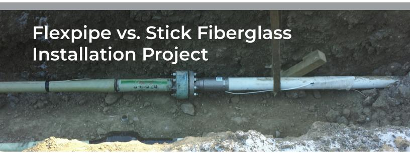
In a side-by-side comparison, Flexpipe Linepipe provided a 20% savings in total installed cost over stick fiberglass.
