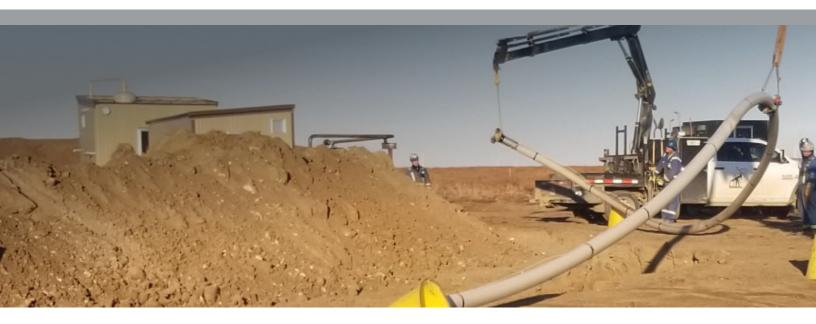
Flexpipe's packaging was an essential part of securing this job. The 12 foot reel height for the new 5" Flexpipe product reaps many benefits. Not only can more product be transported on one truck than other larger diameter pipe manufacturers, but there are also no special permits required on the road. It took Torxen just four trucks of product, with more than 3,200 feet (1,000 meters) of spooled pipe per truck to complete the entire project.
