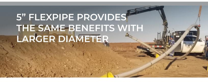
Torxen Resources Ltd. has installed Flexpipe's 3" and 4" spoolable, composite products for the last couple of years because of the ease of installation and its corrosion resistance. In October 2019, Torxen installed 10,500 feet (3,200 meters) of Flexpipe's newest product, 5" Flexpipe High Temperature (5" FP601 HT),
