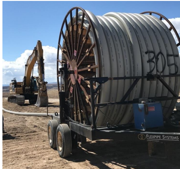
Figure 100: Unspooling from a Moving Deployment Trailer
