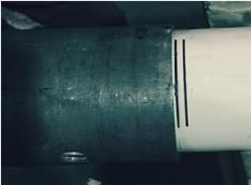
Figure 75: Slide Sleeve Over Pipe
