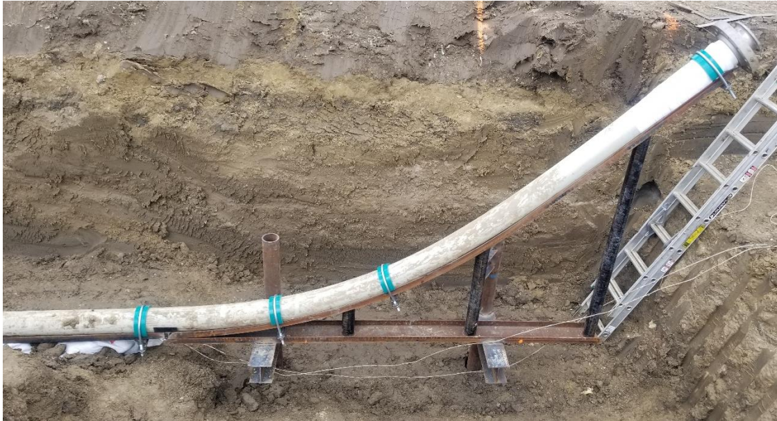
Figure 259: 45-degree Riser Assembly Installation
