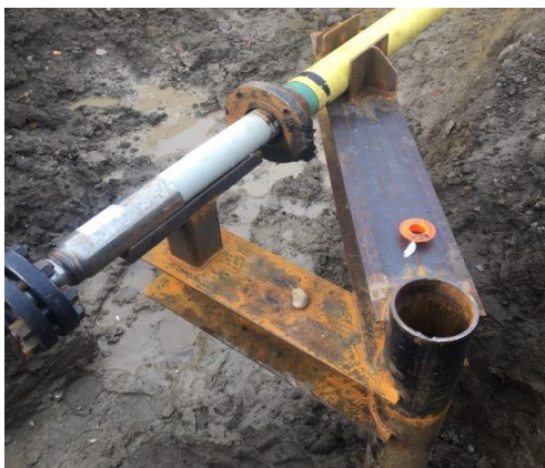
Figure 148: Custom Pipe Anchor Example
