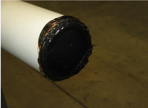
Figure 69: Apply Protective Paste
