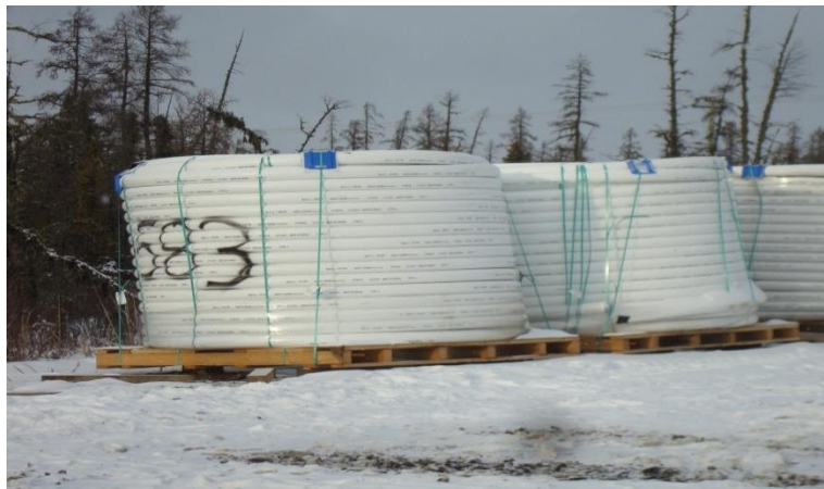
Figure 53: Picture of Winter Storage of Pipe Coils.
