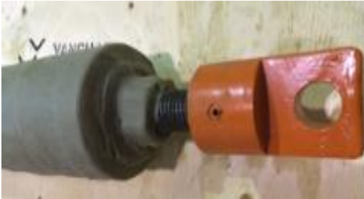
Figure 86: Denso Tape Over Screws and Pipe End
