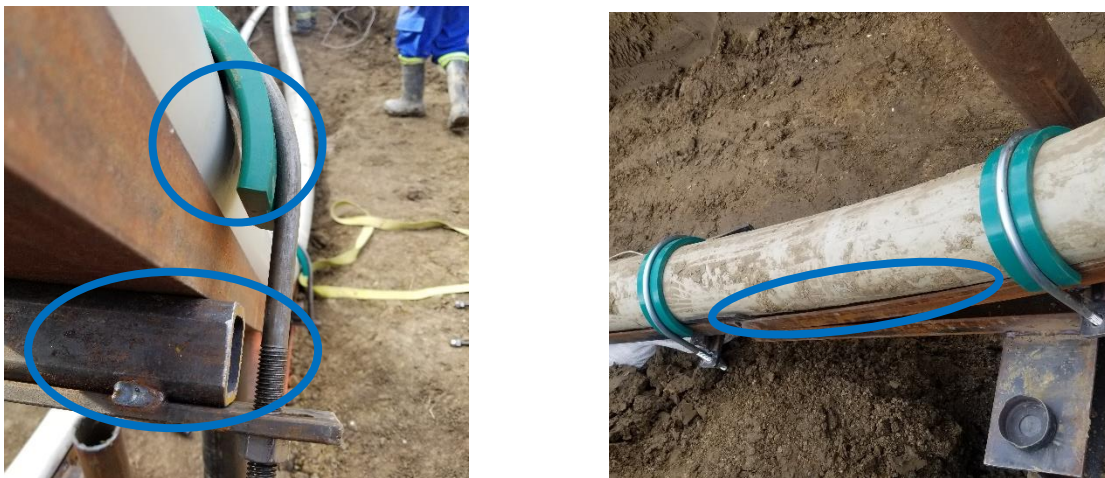
Figure 260: 5" Pipe Gaps and Square Backing
