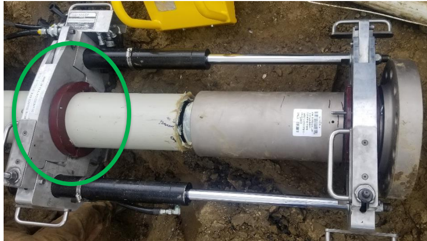
Figure 215: 5" Integrated Pipe Clamp Set for Insertion
