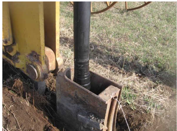
Figure 129: Plowing in a Coupling
