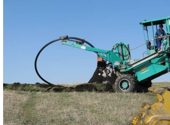
Figure 132: Loop Plowing - Side View
