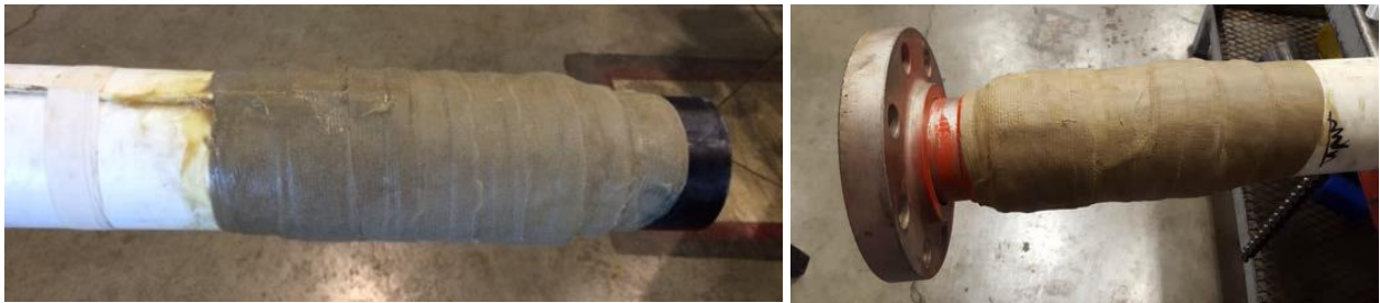
Figure 253: Petrolatum Tape Applied Over Entire Fittings
