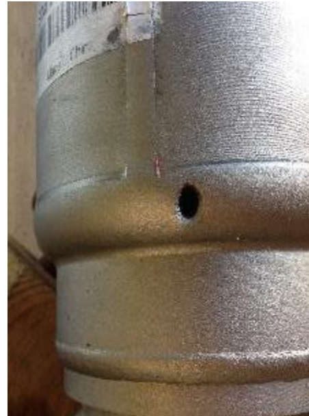
Figure 188: Close-Up of Typical Fitting Vent Hole
