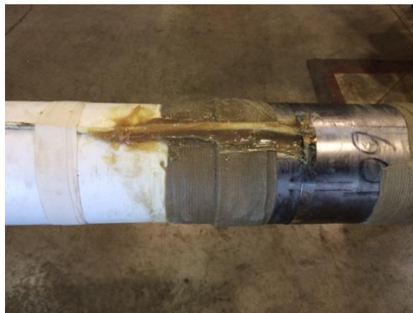
Figure 252: Protective Paste on Anode Wire
