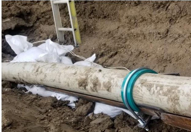
Figure 147: Continuous C-channel and Sandbag Support
