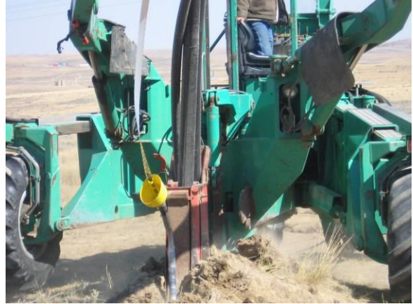
Figure 137: Winch Plowing Multiple Lines
