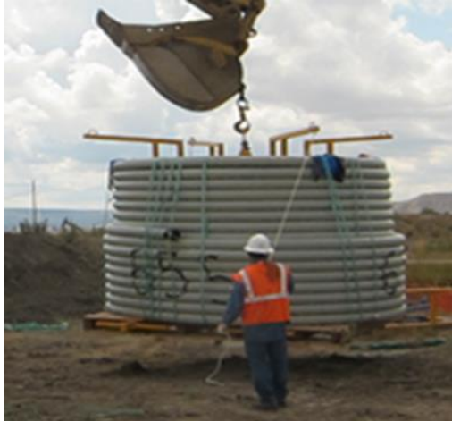
Figure 108: Mounting Coil on Turntable
