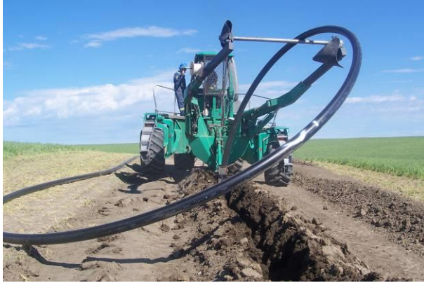
Figure 131: Loop Plowing – Rear View
