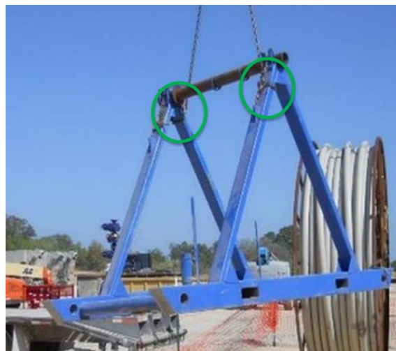
Figure 57: Unloading the A-Frame
