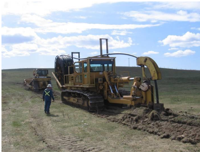
Figure 135: Reverse Bend Plowing with a Mounted Reel
