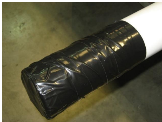
Figure 73: Sealed Pipe End
