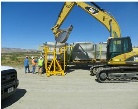
Figure 46: Attaching Device to Backhoe
