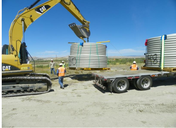
Figure 49: Unloading Coil from Flatbed
