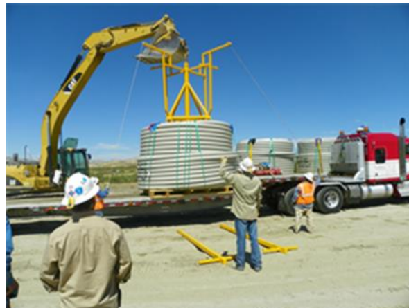
Figure 47: Lowering Device into Coil
