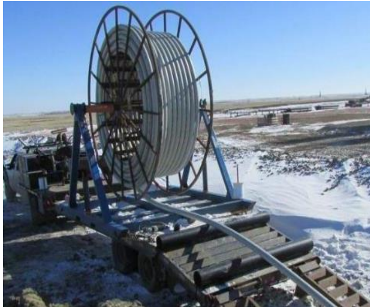
Figure 103: Pulling Pipe from a Stationary A-Frame
