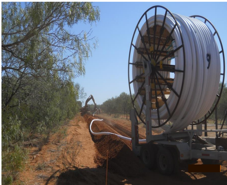
Figure 98: Transporting with a Self-Loading Trailer
