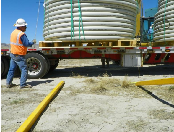
Figure 48: View Through Lifting Pockets
