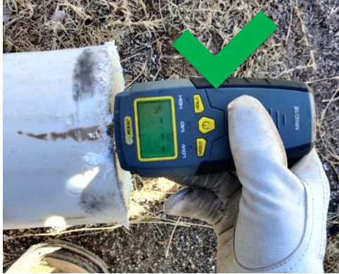
Figure 194: Dry Wetness Measurement
