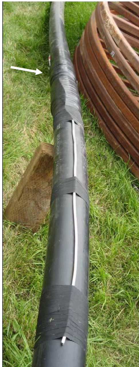
Figure 255: Anode Attached to Fitting for Plowing
