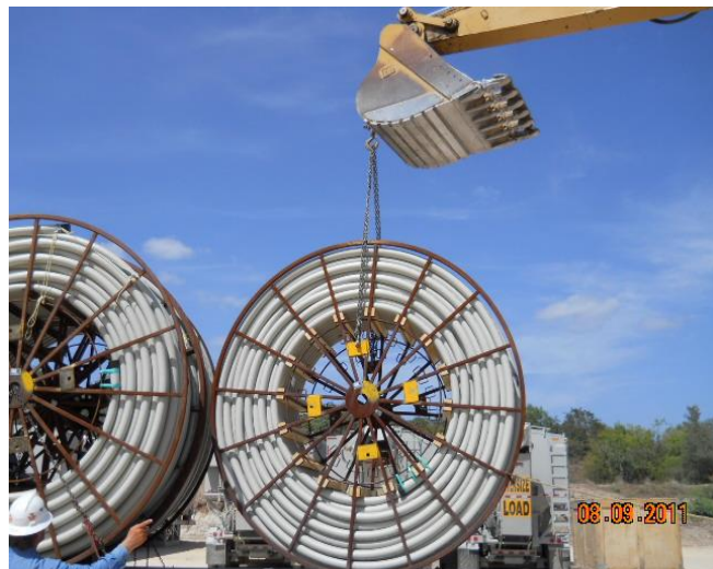
Figure 30: Connected to Lift Plates
