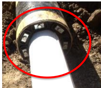
Figure 152: Link-Seal at Casing End – NOT Recommended
