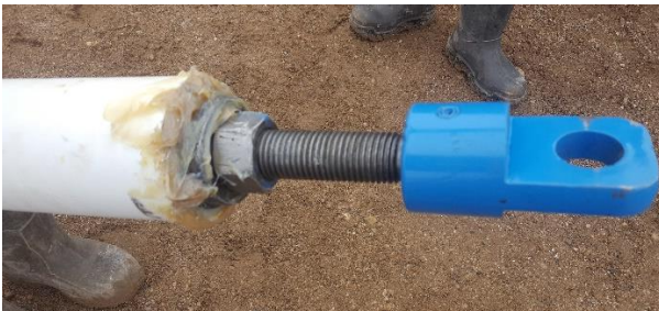
Figure 85: Denso Paste on Pipe End
