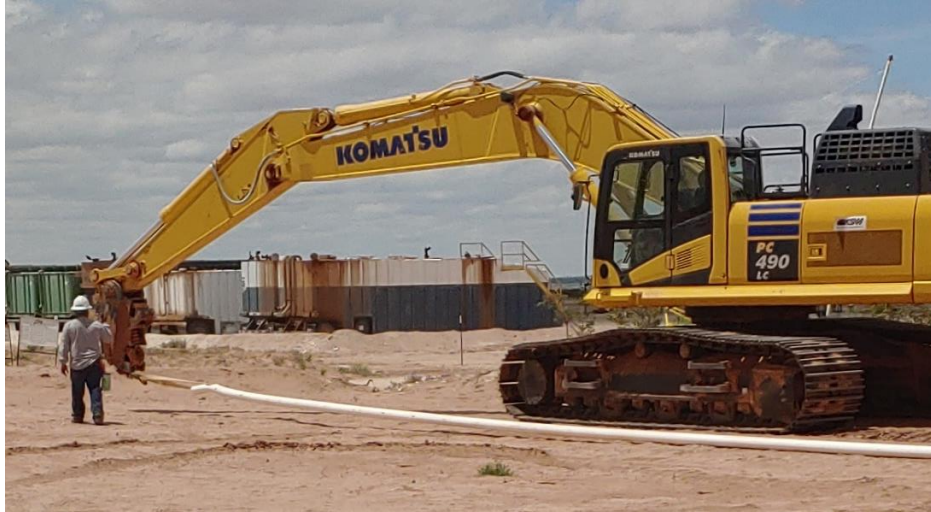
Figure 154: Surface Line Deployment with Strap
