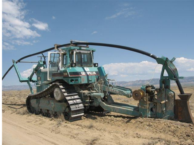
Figure 134: Reverse Bend Plowing with Pre-Strung Pipe
