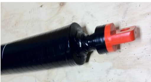
Figure 87: Wrap Pipe and Seal Pipe End
