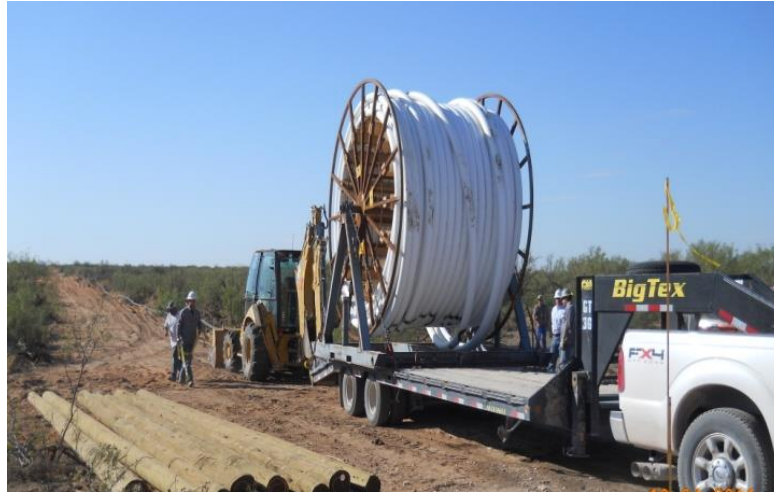
Figure 97: Moving an A-Frame on a Trailer
