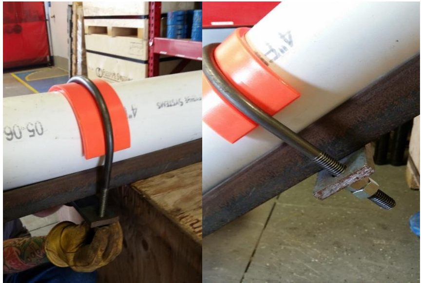
Figure 163: U-Bolt Installation
