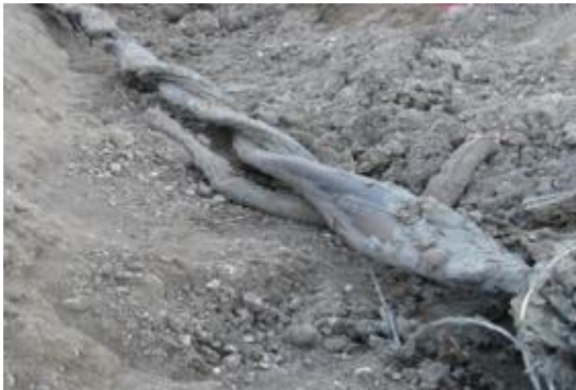
Figure 141: Twisted Pipe from Pull Without Swivels
