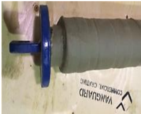
Figure 79: Apply Denso Tape to Protect Fibers
