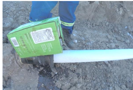
Figure 142: Canola Oil Lubrication in Liner Pull
