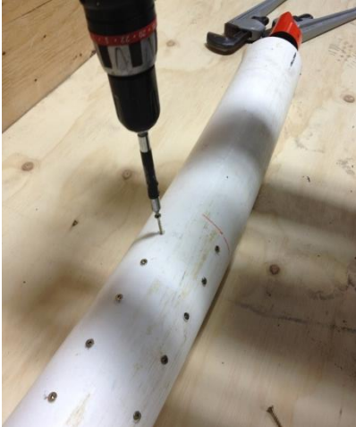
Figure 84: Securing Pipe with Screws
