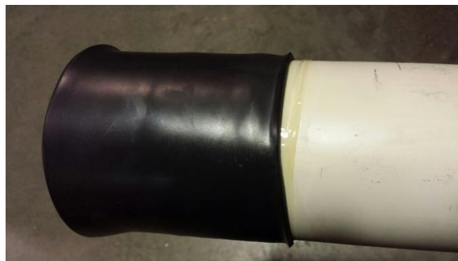
Figure 28: Heat Shrink Cap Installed On Pipe End
