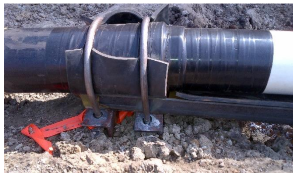
Figure 149: C-channel Secured by U-Bolts
