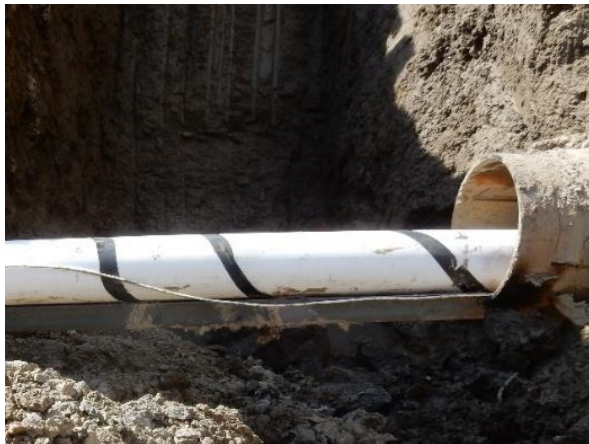
Figure 144: C-channel Welded to Casing Exit
