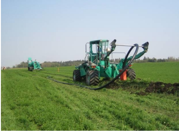
Figure 136: Winch Plowing
