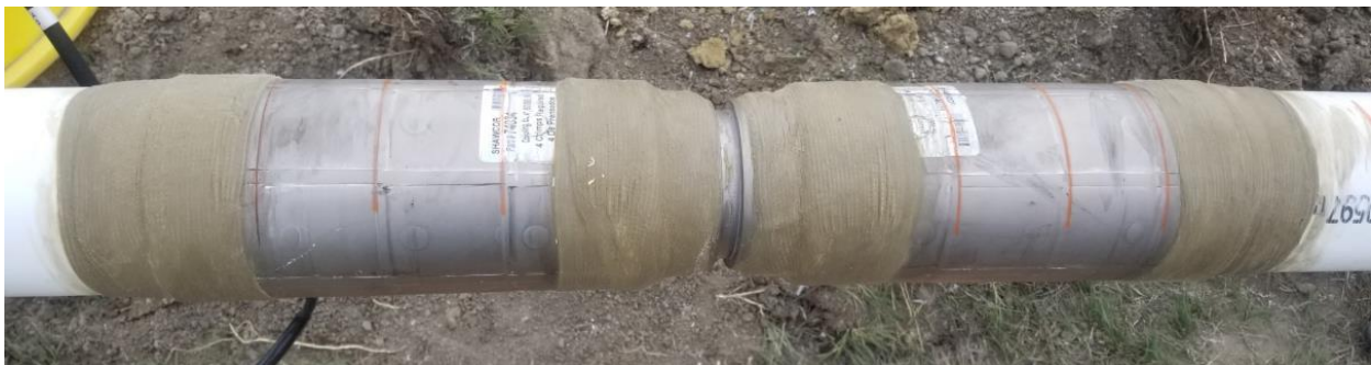
Figure 249: Wrapped Vent Hole Area and Sleeve Ends
