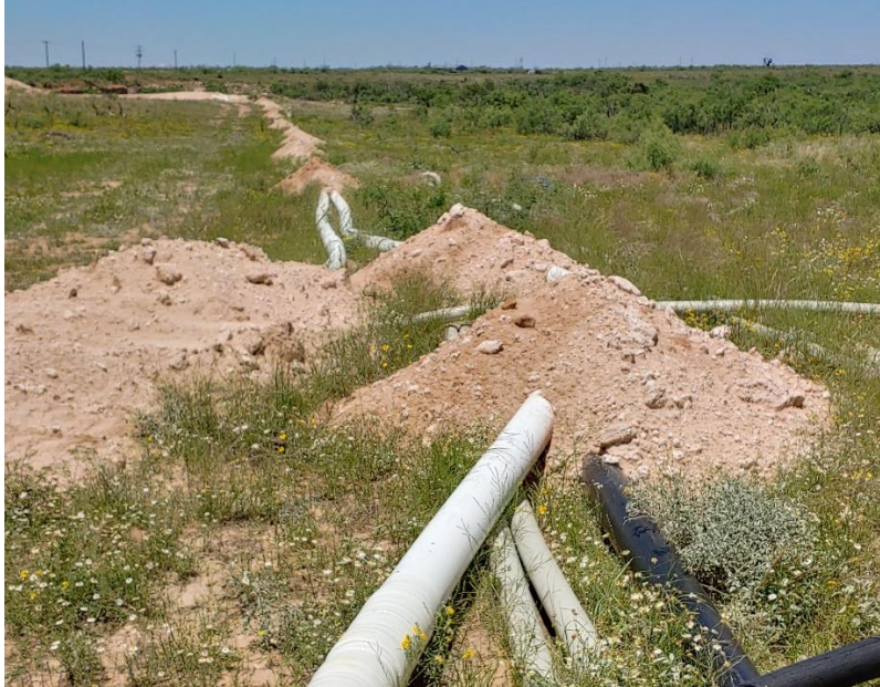
Figure 155: Dirt Piles Used For Pipe Restraint
