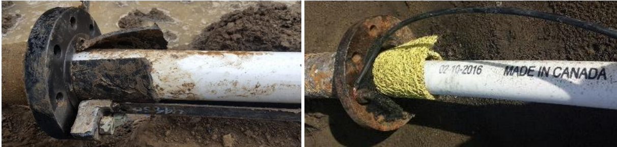
Figure 150: Padding Examples At Casing Edges
