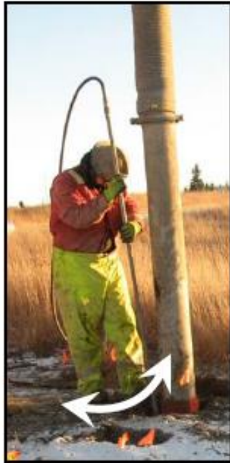
Figure 267: Hydrovac Exposing a Buried Pipeline
