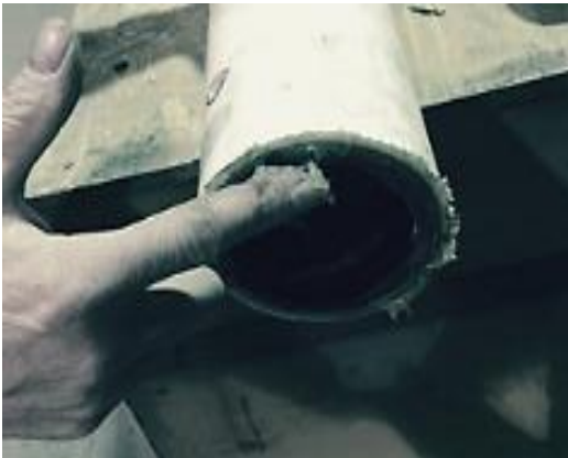
Figure 77: Apply Paste to Protect Fibers
