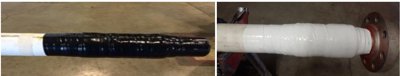
Figure 254: Fully Wrapped Fittings
