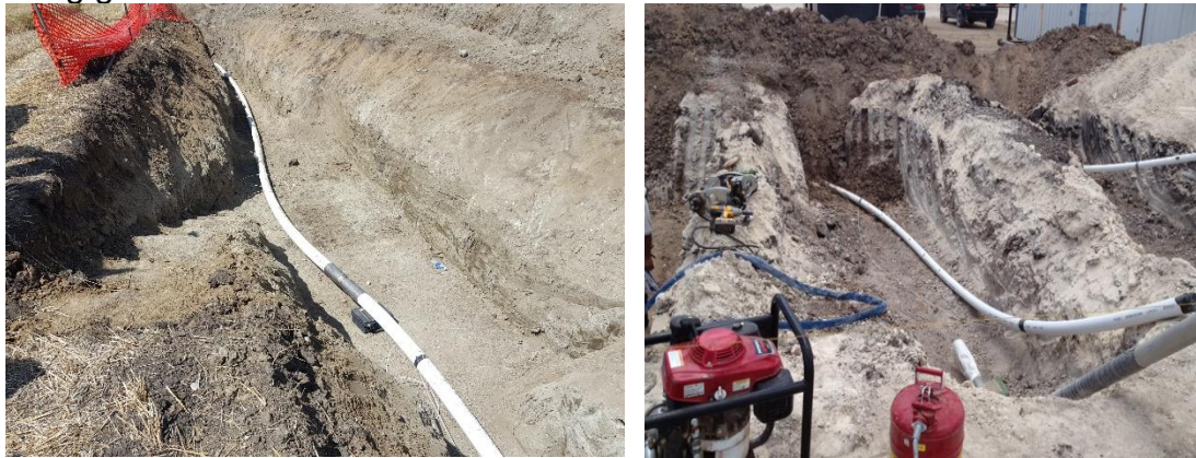
Figure 125: Crimping a Fitting in the Ditch
