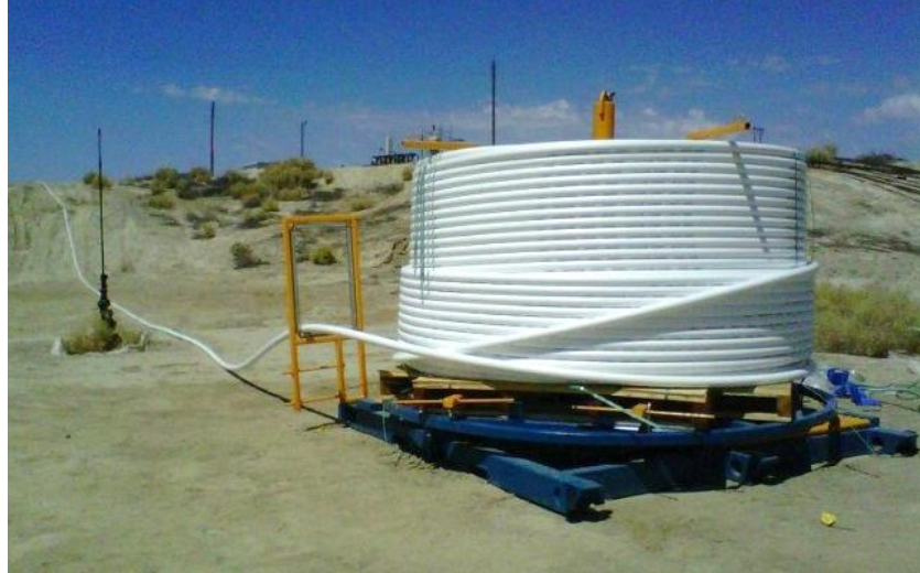
Figure 114: Coil Being Deployed
