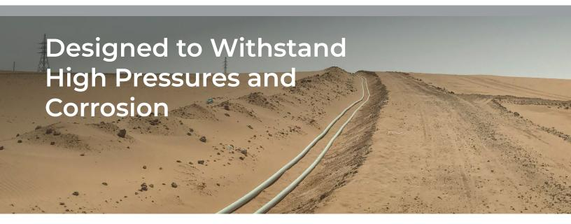
Constructed from a winning combination of high-density polyethylene, helically wound epoxy-free dry fiberglass and a protective outer jacket, Flexpipe products are safe to install thanks to smaller crew sizes and less heavy equipment requirements.
