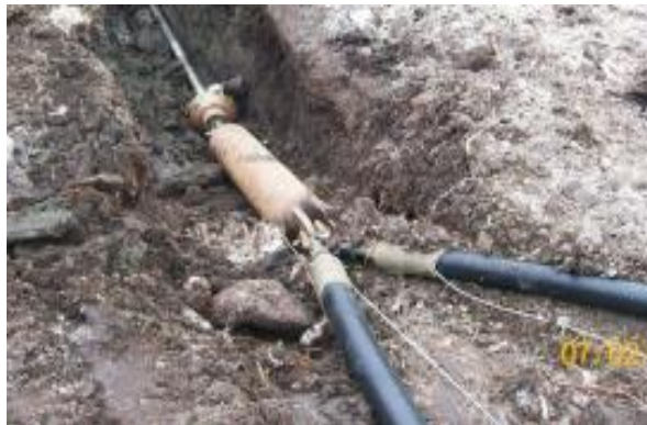
Figure 2: Swivel Heads for Multiple Lines
