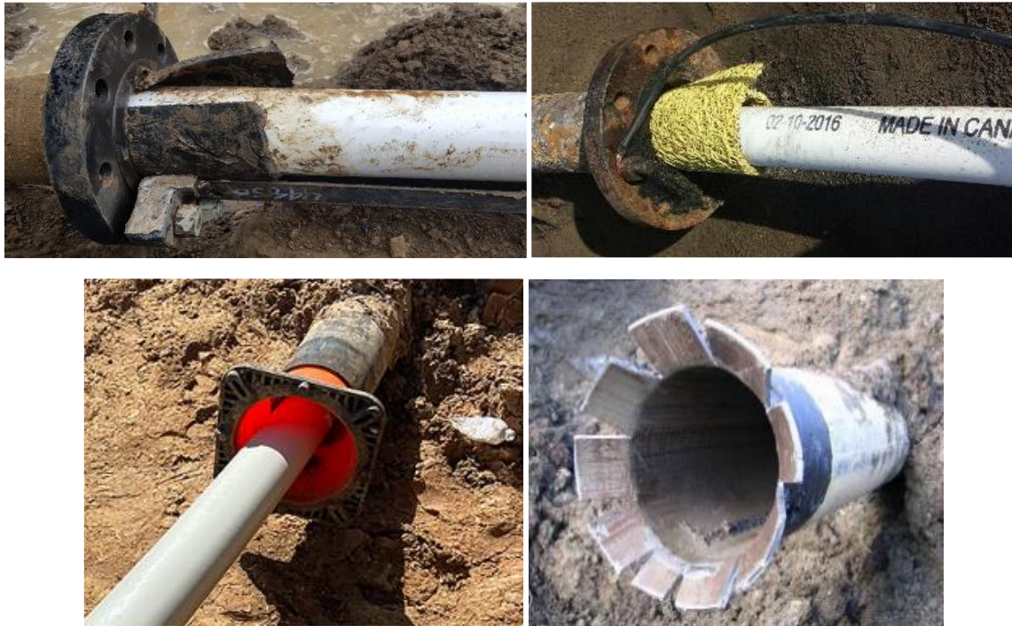
Figure 12: Examples of Casing Edge Protection
