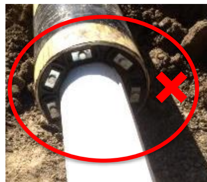
Figure 13: Link-Seal at Casing End
