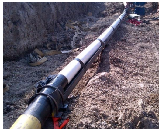
Figure 7: Continuous C-Channel Support
