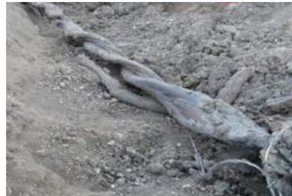
Figure 3: Twisted Pipe Pulled Without Swivels
