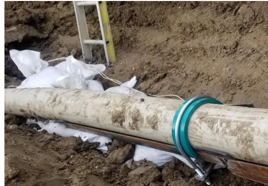
Figure 9: C-Channel & Sandbags Continuous Support
