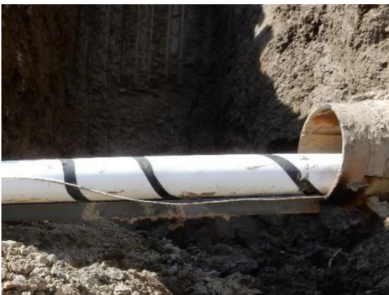
Figure 6: C-Channel Welded to Casing Exit
