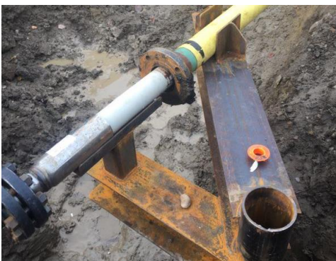
Figure 10: Custom Pipe Anchor Example
