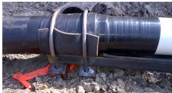
Figure 11: C-Channel Secured to Casing by U-Bolts
