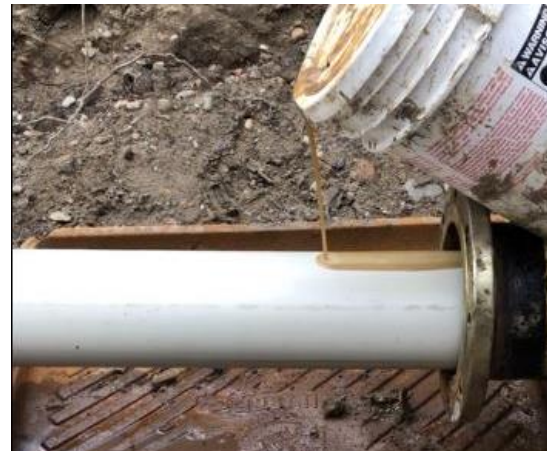
Figure 4: Lubrication for Liner Pull
