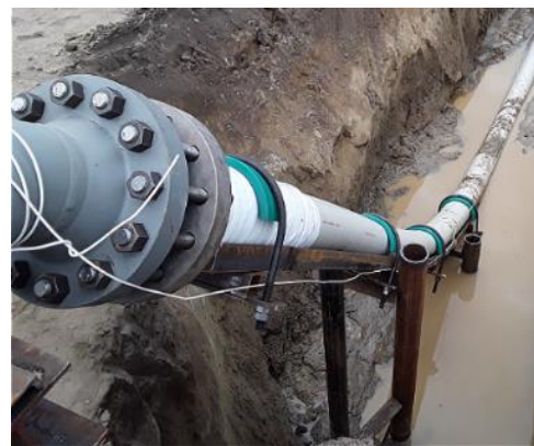
Figure 36: Square backing tubing and gap between the plastic half-moon and the pipe (left). Gap between the pipe and C-channel (right).
