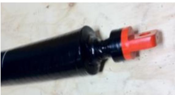
Figure 12: Wrap Pipe and Seal Pipe End
