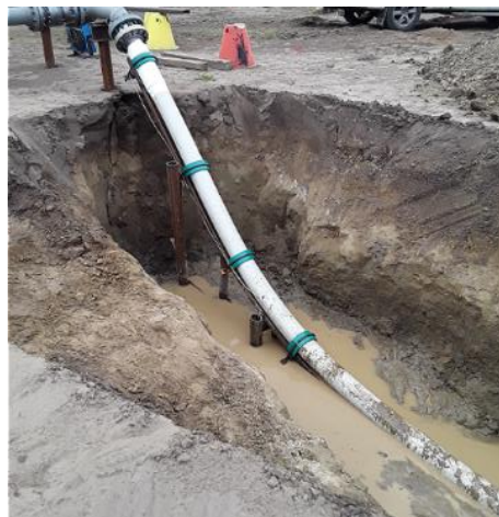
Figure 35: 6" FP601 HT installed into a 45° riser chute
