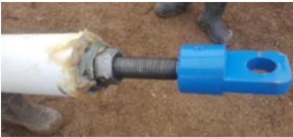
Figure 10: Protective Paste on Pipe End
