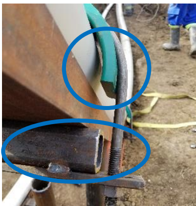
Figure 36: Square backing tubing and gap between the plastic half-moon and the pipe (left). Gap between the pipe and C-channel (right).
