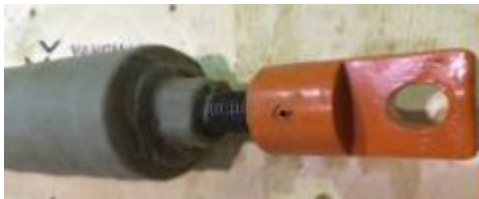
Figure 11: Petrolatum Tape Over Screws and Pipe End
