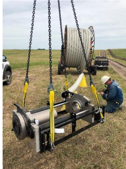
Figure 27: Mandrel Insertion Press suspended by chain-slings.
