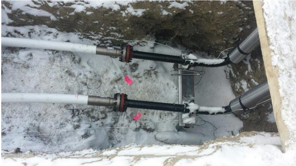
Figure 2: Flexpipe connected to a rigid (steel) pipe riser
