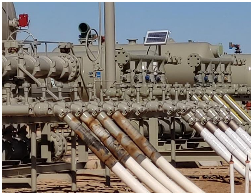
Figure 6: Acceptable surface pipeline support
