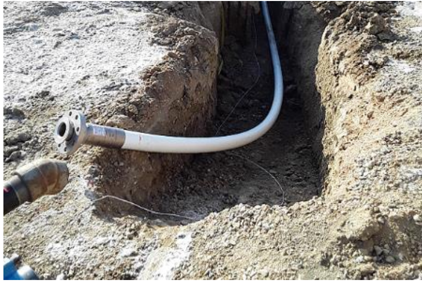
Figure 3: Properly supported virgin soil riser
