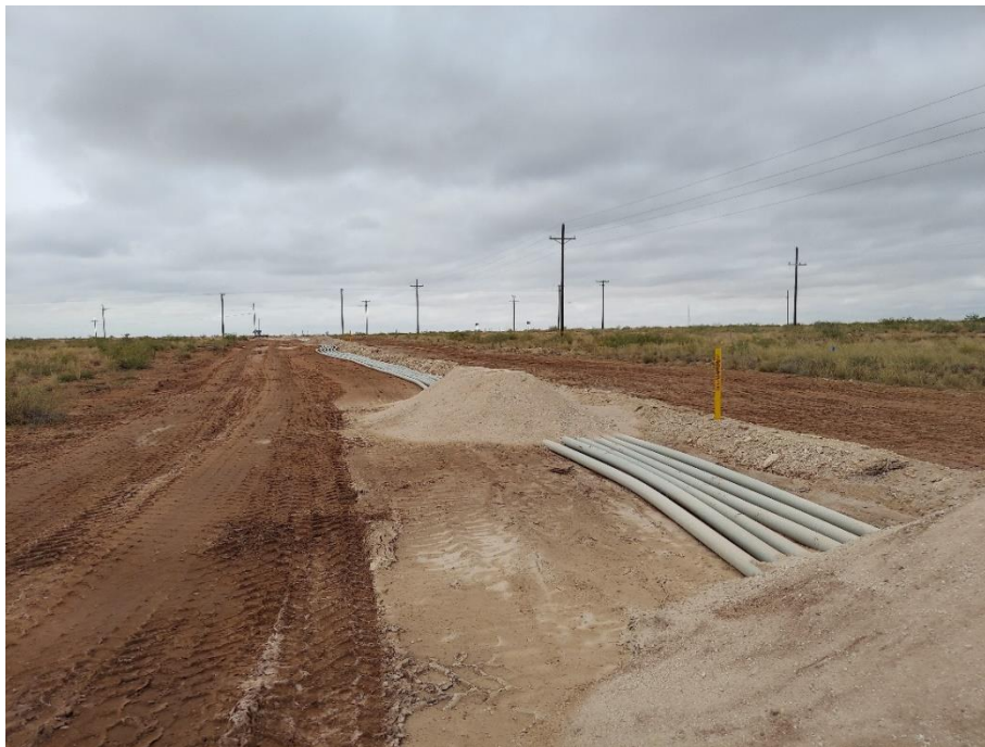
Figure 16: Anchoring the Surface Pipeline after Pressure Testing using Sand Piles
