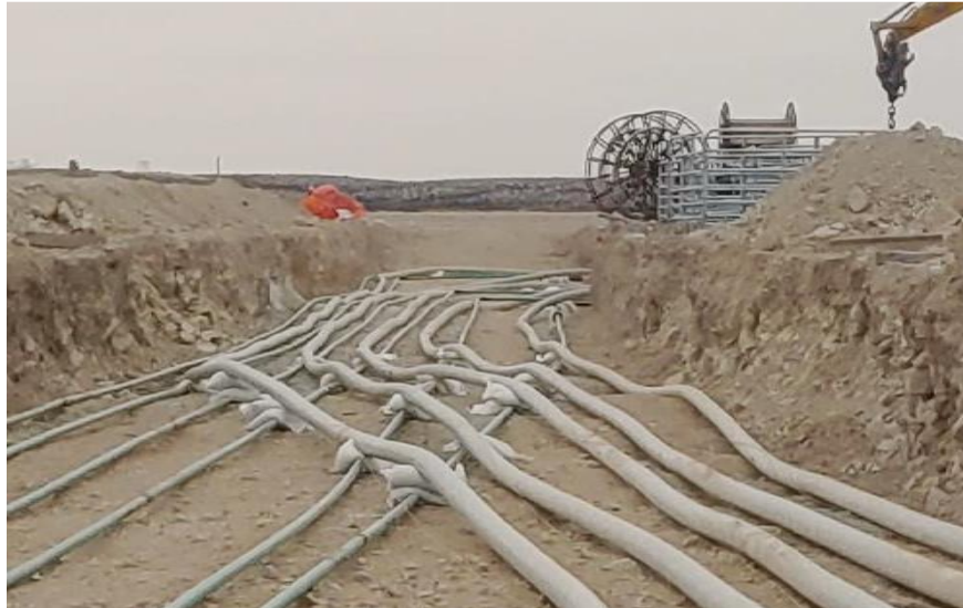
Figure 7: Flexpipe Line Crossings Protected by Sandbags and Sand Piles
