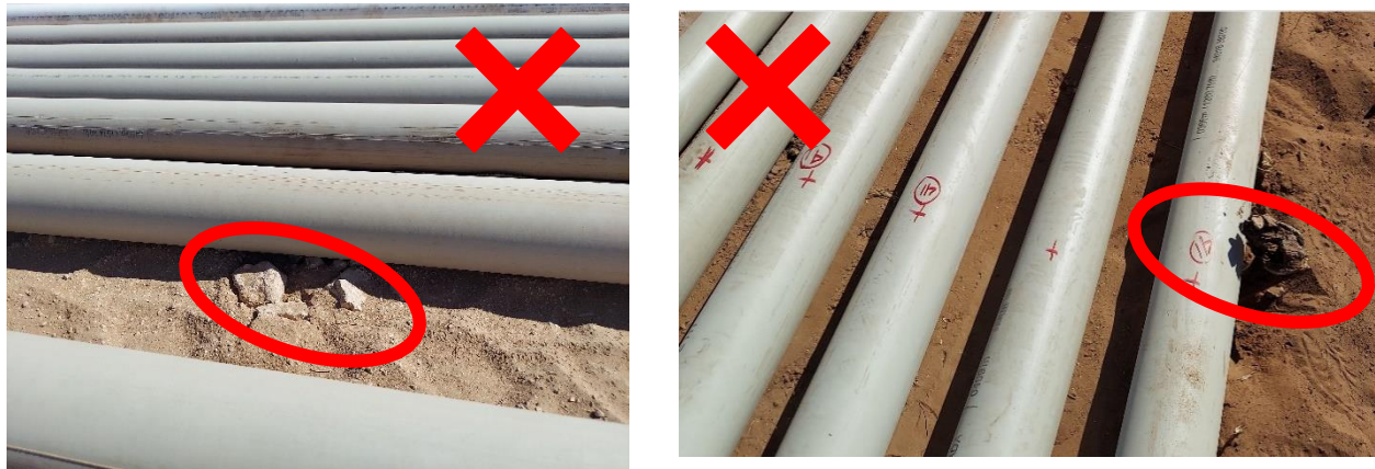
Figure 13: Remove any Large Rocks or Other Objects to Avoid External Damage
