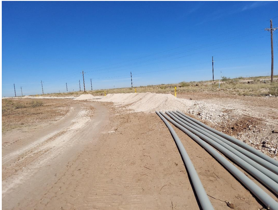
Figure 17: Pipeline Curve Covered with Sand Piles after the Pressure Test
