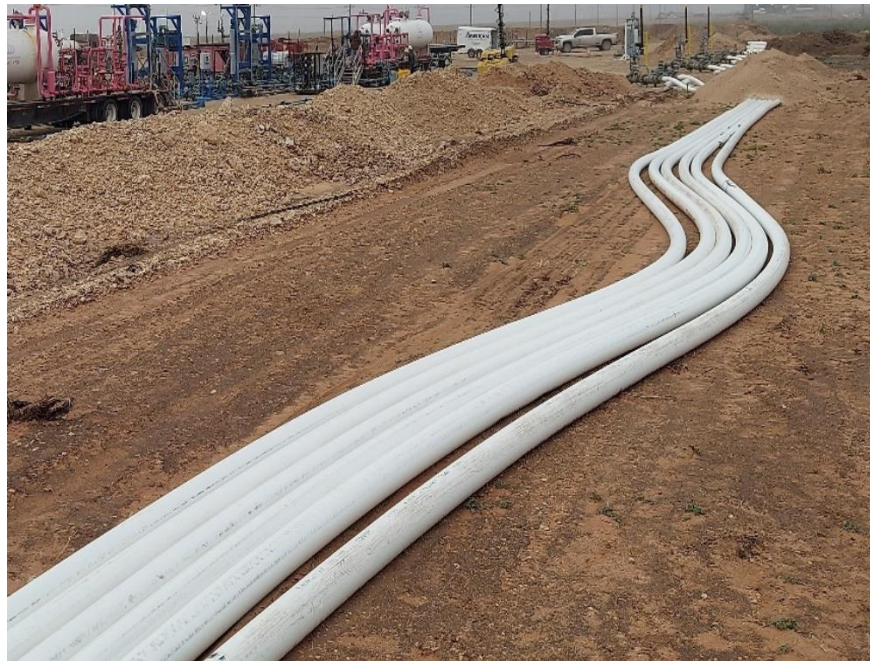
Figure 1: Expected Lateral Displacement after Axial Expansion due to Pressure and Temperature Fluctuations
