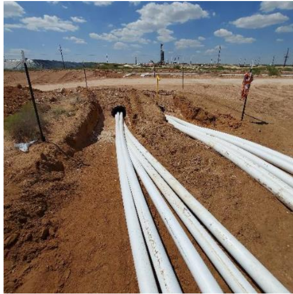
Figure 5: Cased Crossings for Flexpipe Spoolable Products
