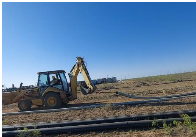
Figure 9: Surface Pipeline Deployment Using a Swivel
