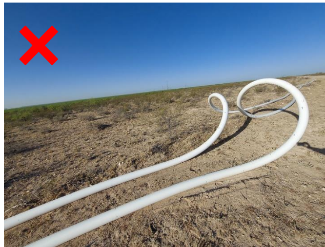
Figure 15: The Risk of Forming Twisted Sections Increases When the Pipe is not Allowed to Rotate to a Neutral Position
