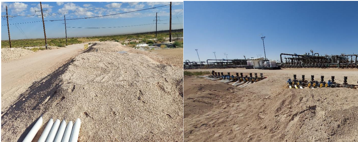
Figure 2: Sand Piles at Pipeline Entry to Facilities
