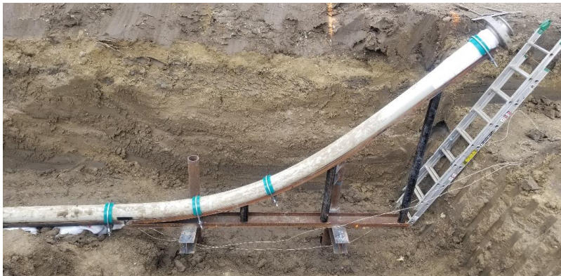
Figure 15: 5" FP601 HT installed into a 45° riser chute
