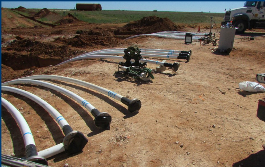
Figure 1. High CO 2 Gathering Lines During Construction
